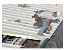
\*Between two blankets, jointing together with stapler binding in facing long edge side.
