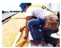
\*Pay attention to keep tensioning of the glass woll, align, joint spaces between blankets, when lengthways needs to jointing, the joiner should fix up in purline.
