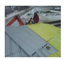
\*Install roof color steel board,take off the special clamp in eaves two sides, seal it with the reserved 20cm facing.
